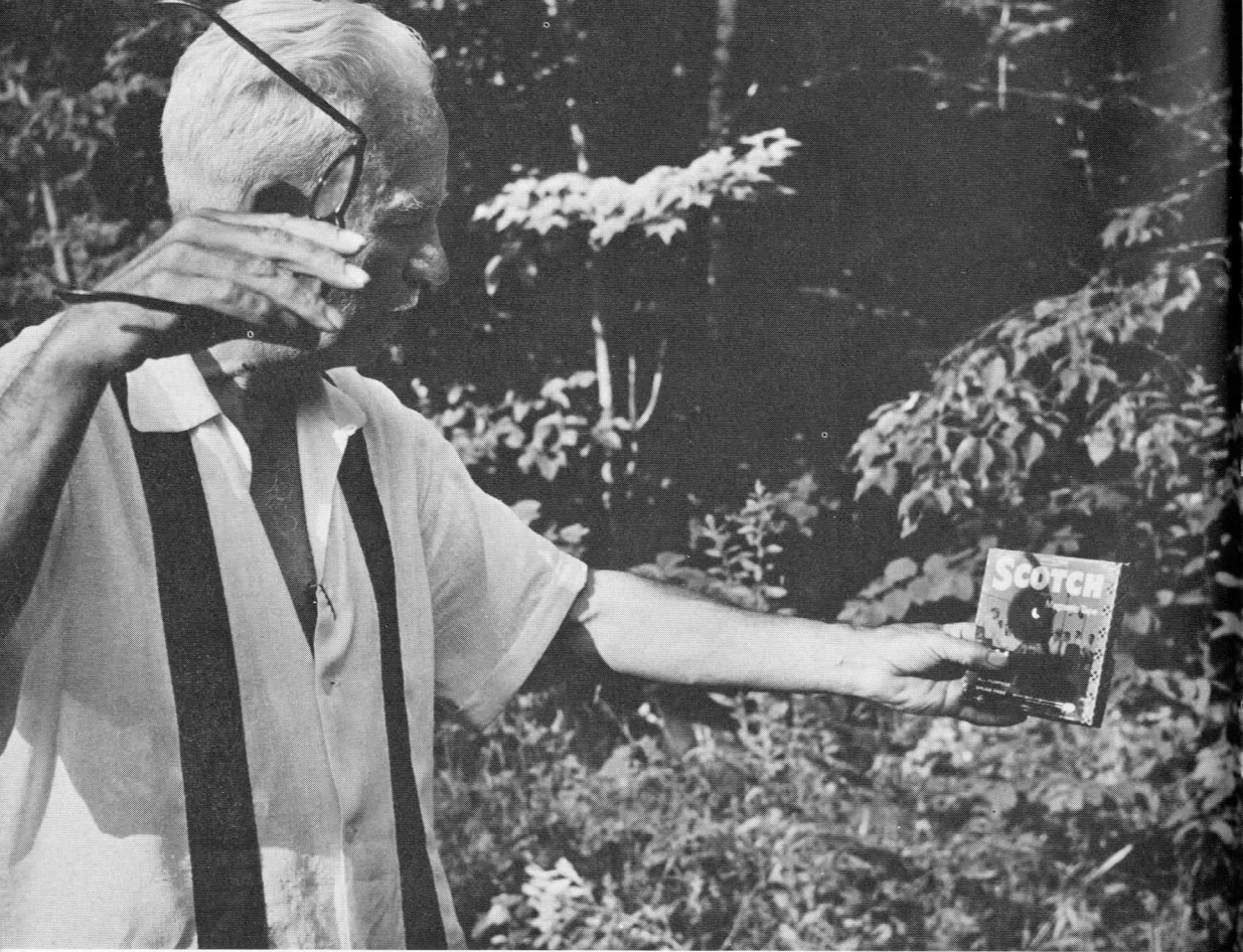
Figure 3. Using a 30-centimeter lens to project the bright image of the partly-eclipsed sun on a box of magnetic tape, the senior author follows the progress of the eclipse.
